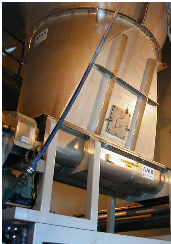
Figure 1 shows the new AJAX hopper and triple screw feeder.
